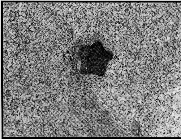
Detail of the star-shaped hole drilled in the rock near Bay Tree Spring.
